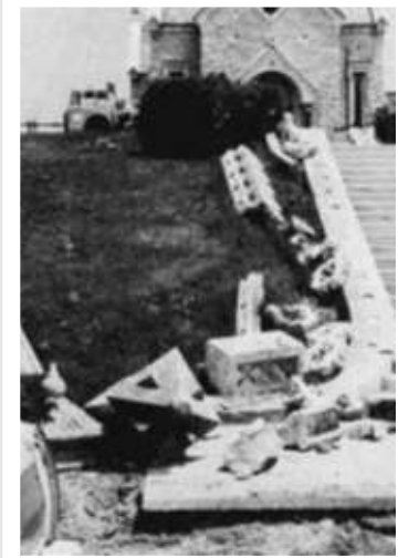
Before. Rails destroyed by a tornado
