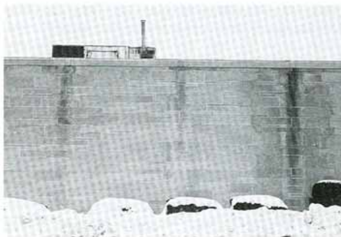
Leaking connections in this metal coping collect water and dirt which flood over the stone below in a concentrated flow.
